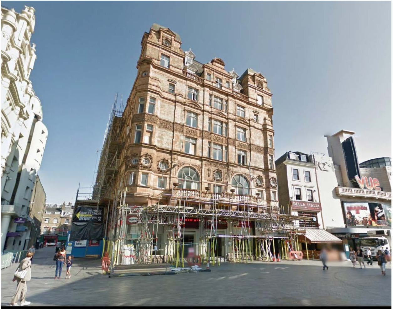
The front elevation of Victory House facing onto Leicester Square
